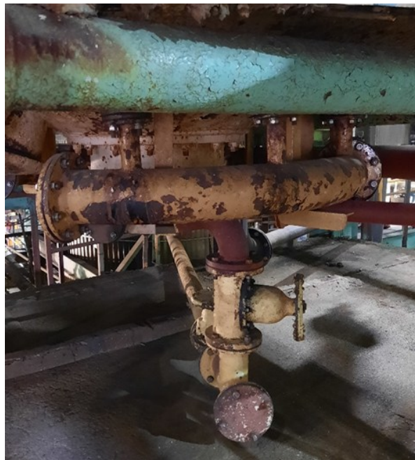
Figure 19. Evaporator external feed ring with feed risers
