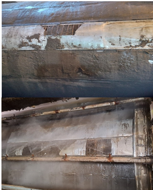
Figure 18. Poor filter cake formation with the damaged screen area commonly observed in the factories
