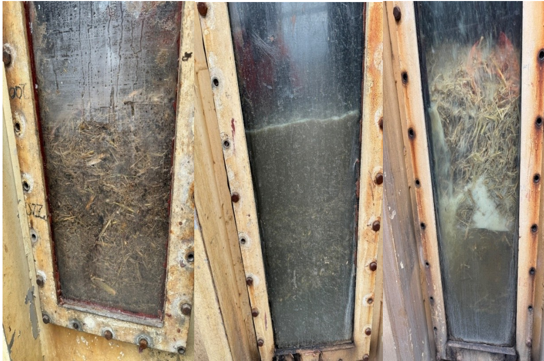
Figure 7. A combination of photographs taken of one diffuser, showing uneven bed levels with flooded and dry beds, as commonly seen during the visits
