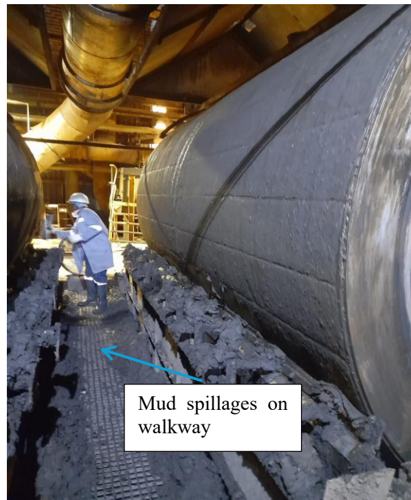
Figure 8. Oliver filters in operation at Simunye sugar mill.
