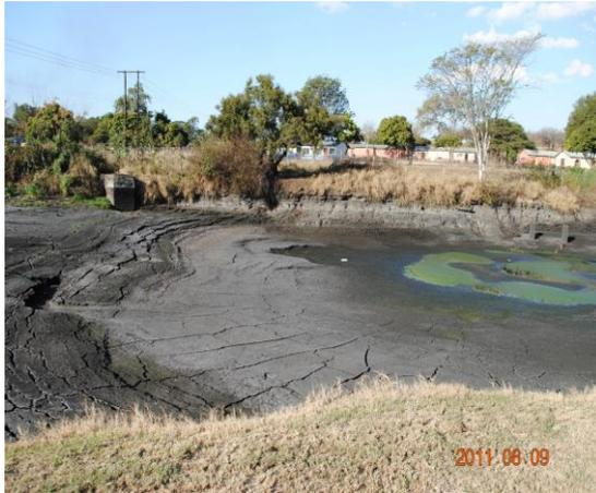
**Figure 2. Dam 1 drying out for desludging.**
