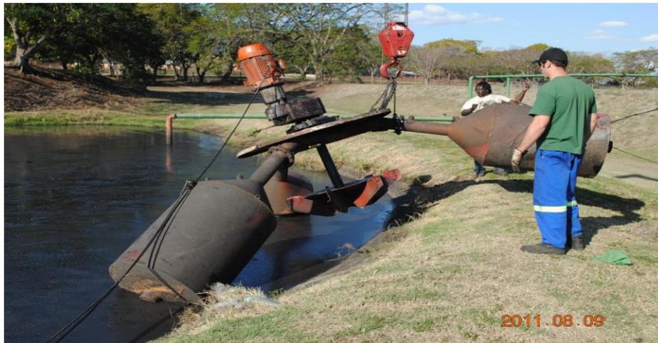
**Figure 10. Floating aerator being removed for refurbishment.**
