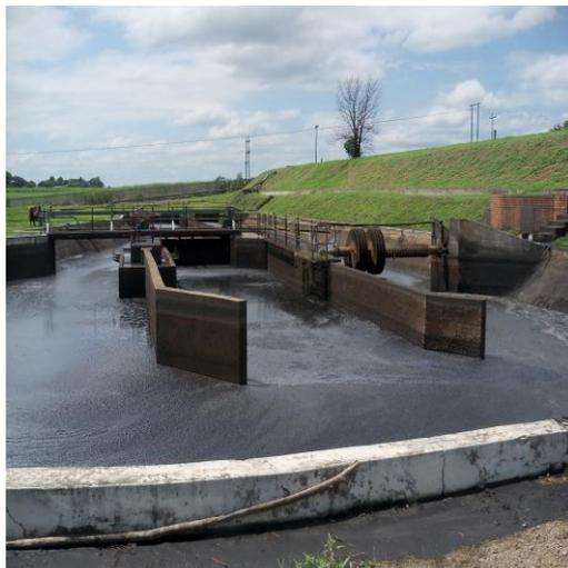
**Figure 6. Ash-filled Pasveer ditch.**
