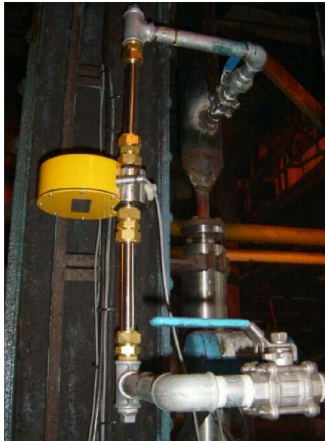
**Figure 1. The SRI Sucrose Analyser (yellow unit) installed in Darnall sugar mill, monitoring syrup.**
