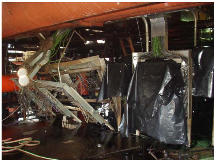
**Figure 7. Damage to control panels.**
