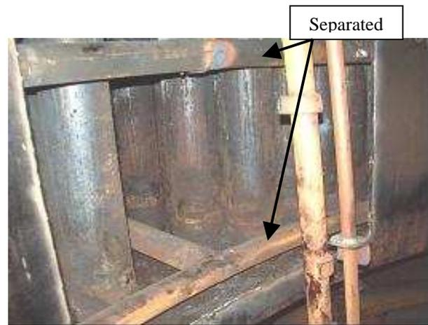
**Figure 2. Pipes for light and heavy incondensable gases separated.**
