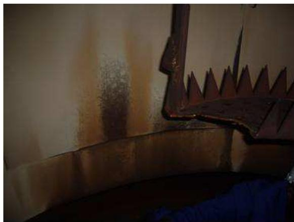
Figure 4. Broken section of the condenser rainmaker.
