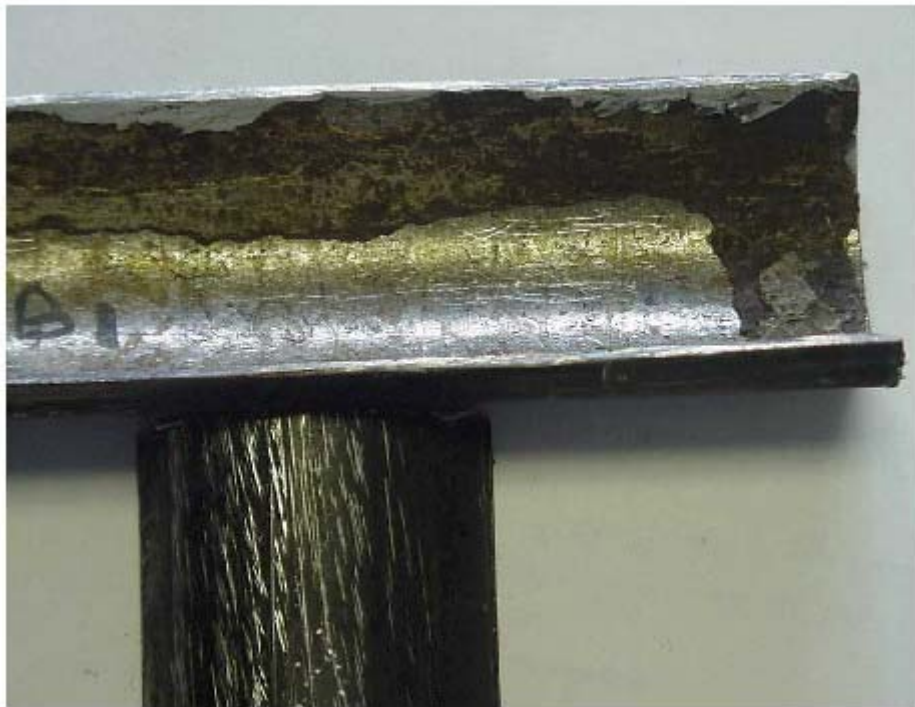
Figure 6. A section of tube showing scale that was not removed by mechanical cleaning.
