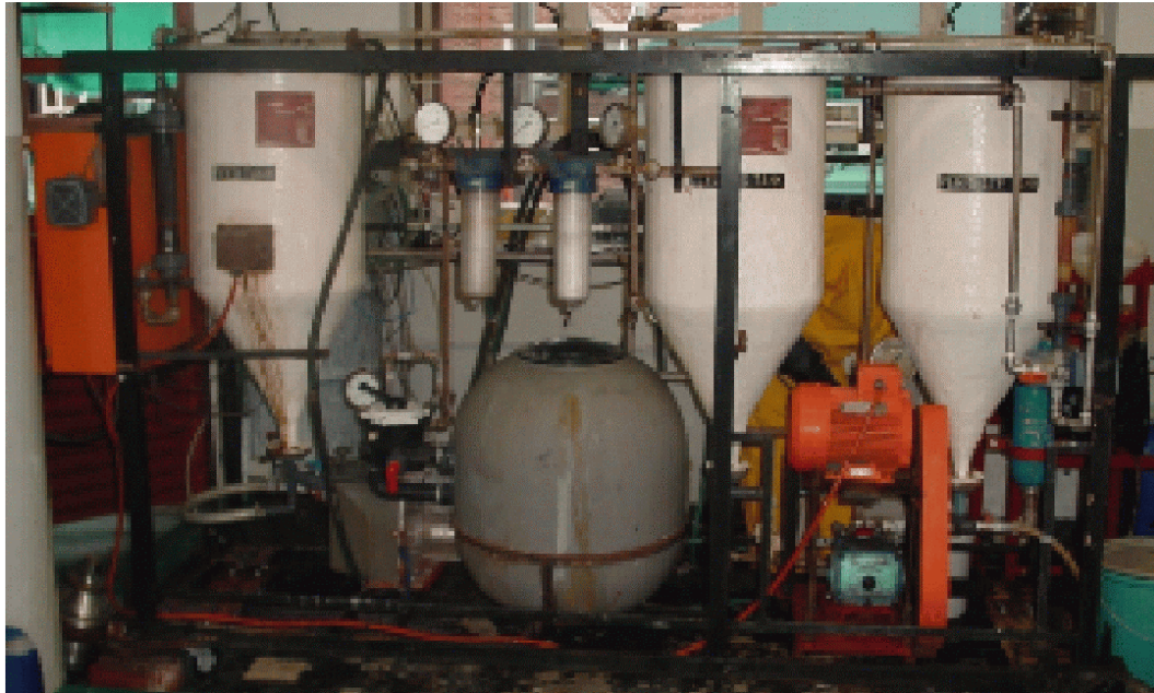
Figure 1. The membrane filtration rig.
