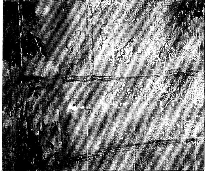
FIGURE 5 Batch pan steam chest inlet internal before epoxy coating.
