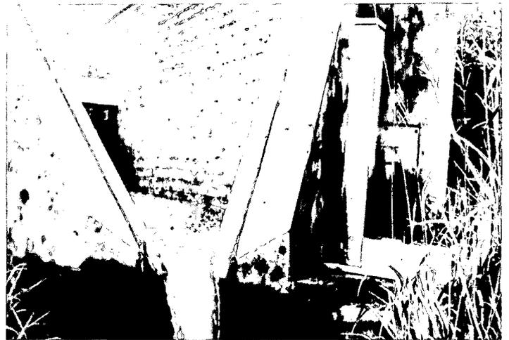
**FIGURE 6** Final discharge of runoff through the mouth of the H flume in catchment 101.
