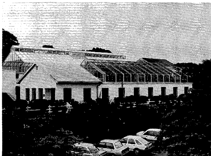
FIGURE 2 The new quarantine building at Mount Edgecombe was opened in 1984.
