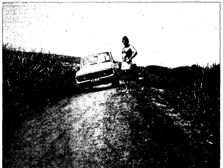
FIGURE 11 Terrace road showing the backslope into the hillside and the waterbearing channel.
