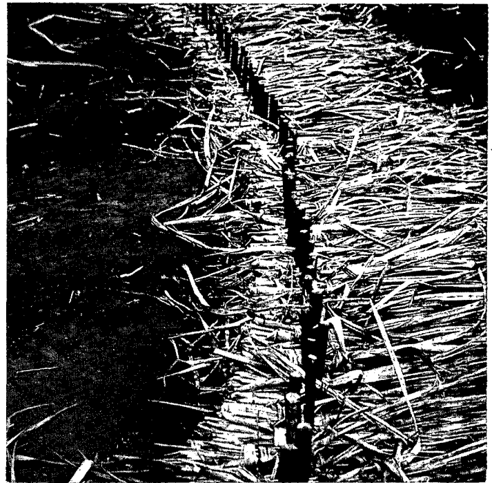
FIGURE 10 Close-up of a revette in a newly constructed waterway, consisting of bundles of cane tops pegged into the ground with their butts pointing up-slope.
