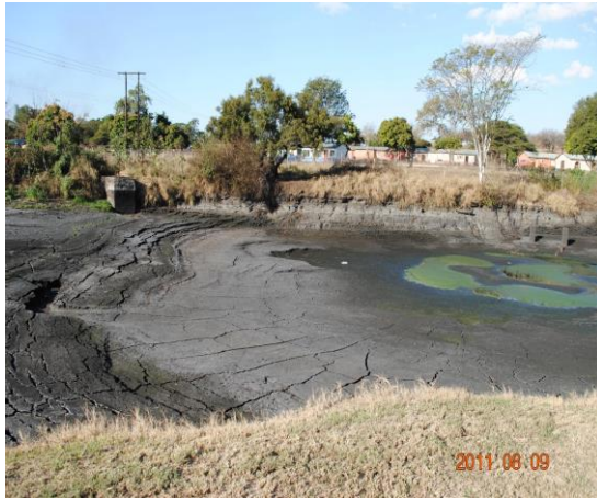
Figure 2. Dam 1 drying out for desludging.
