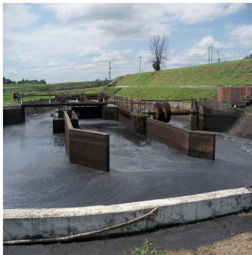
Figure 6. Ash-filled Pasveer ditch.
