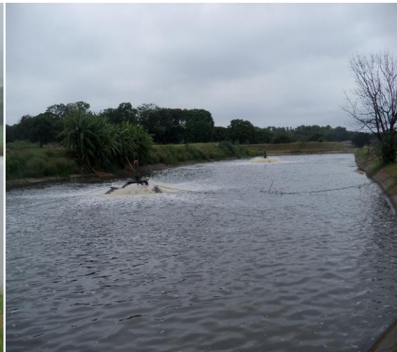
Figure 5. Dam 3 with two floating aerators instead of three aerators.
