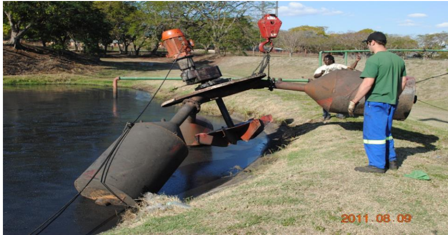
Figure 10. Floating aerator being removed for refurbishment.
