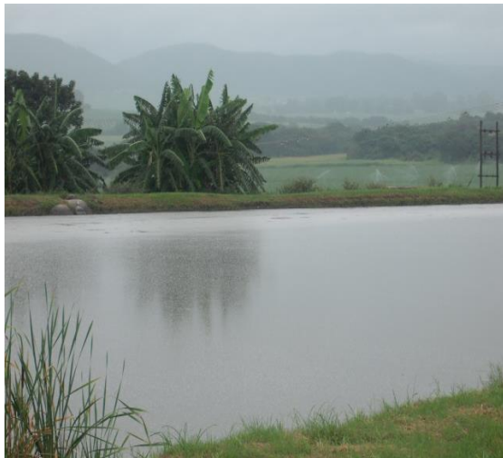
Figure 4. Anaerobic pond, Dam 2, indicating poor anaerobic activity.
