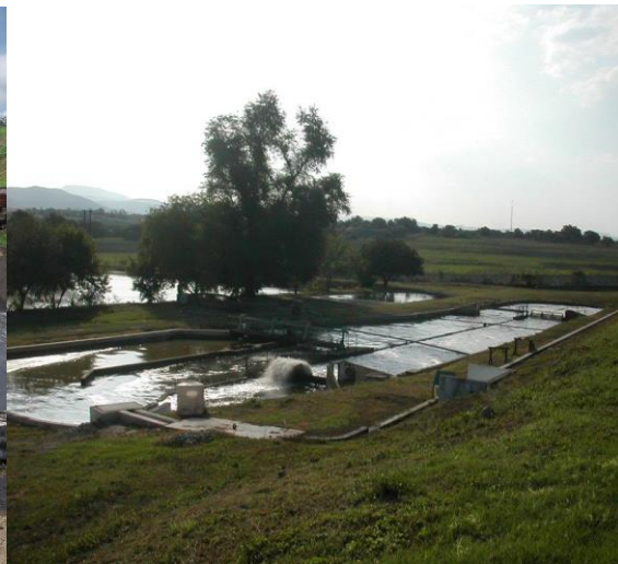
Figure 7. Dam 4 showing poor aeration with damaged aerator.
