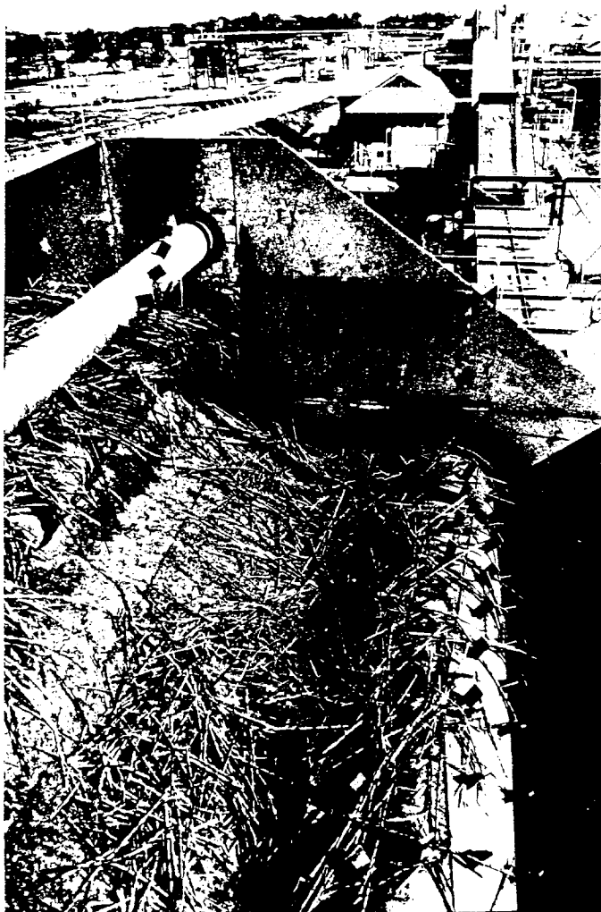
FIGURE 2 A view of the rock removal system showing the feeder table with scratcher, inclined side table and tined drum. The cane preparation line can be seen in the background.
