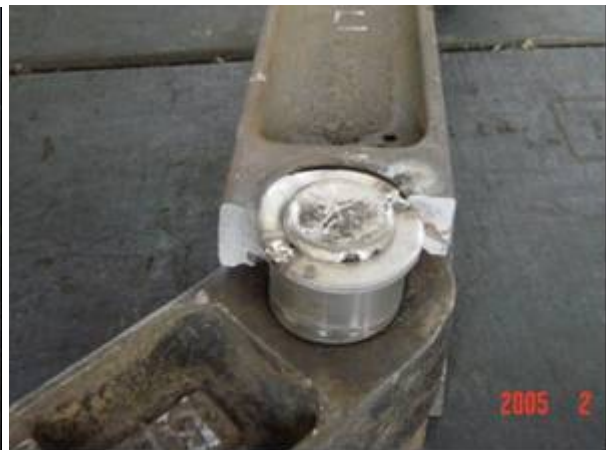
Figure 6. Mating failed section to Figure 5.
