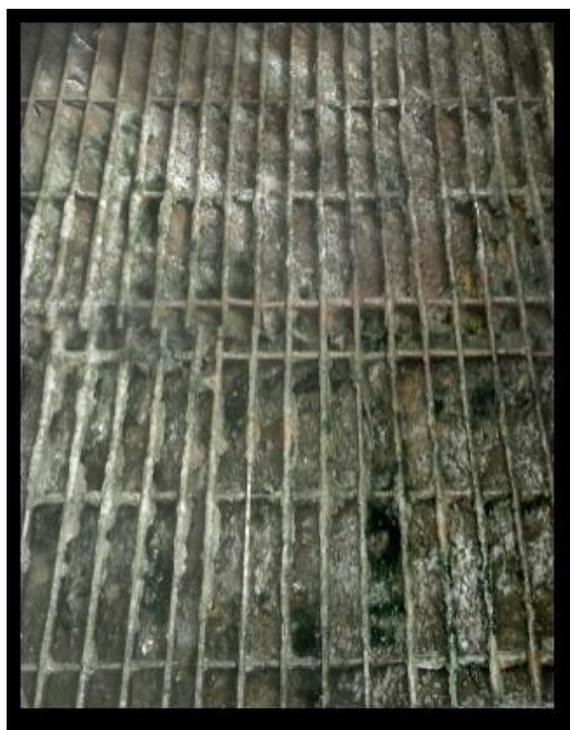
**Figure 8. Organic growth on cooling tower drift eliminators.**
