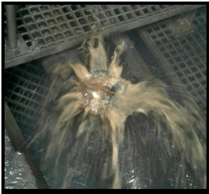
**Figure 4. 'Clean' water application up sprayer fitted to 'dirty' water cooling tower.**
