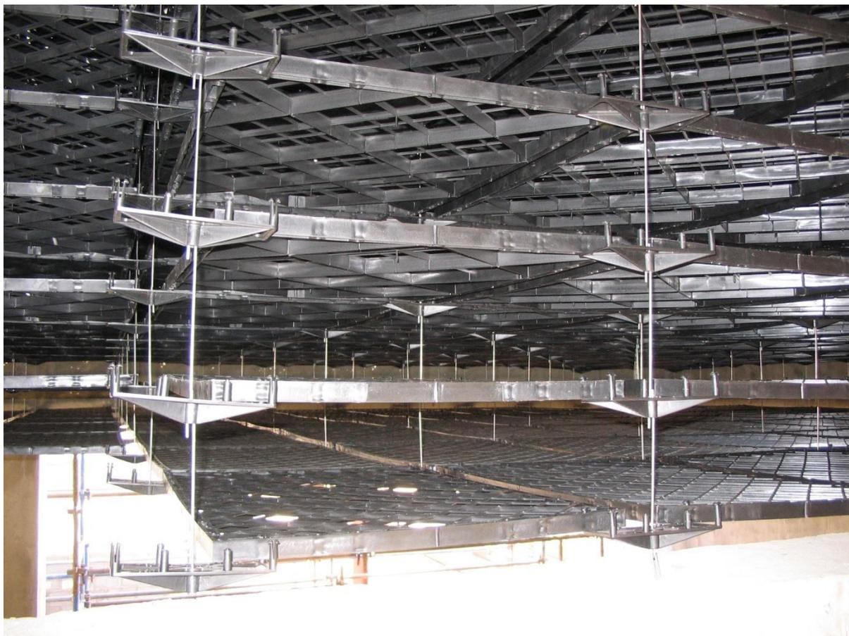
**Figure 5. Splash grid fill (Industrial Water Cooling Pty Ltd).**
